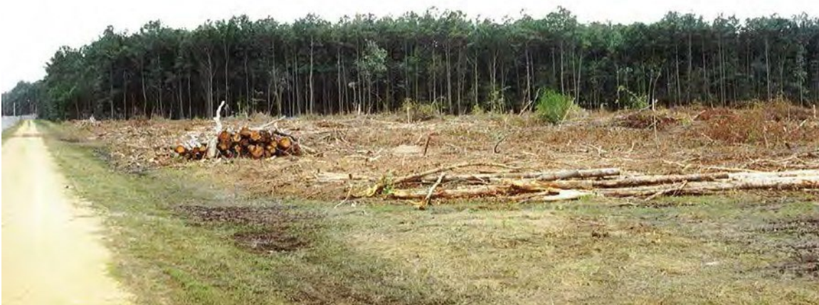
Runway clearing project at Webster Outlying Field: An Illustration of the Management Practices and Prescriptions (MPPs).
