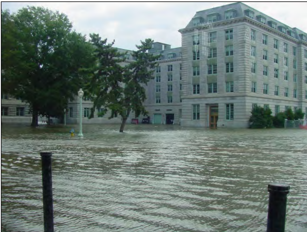
Figure 1-4 Flooding after Hurricane Isabel 2003, Photo II
