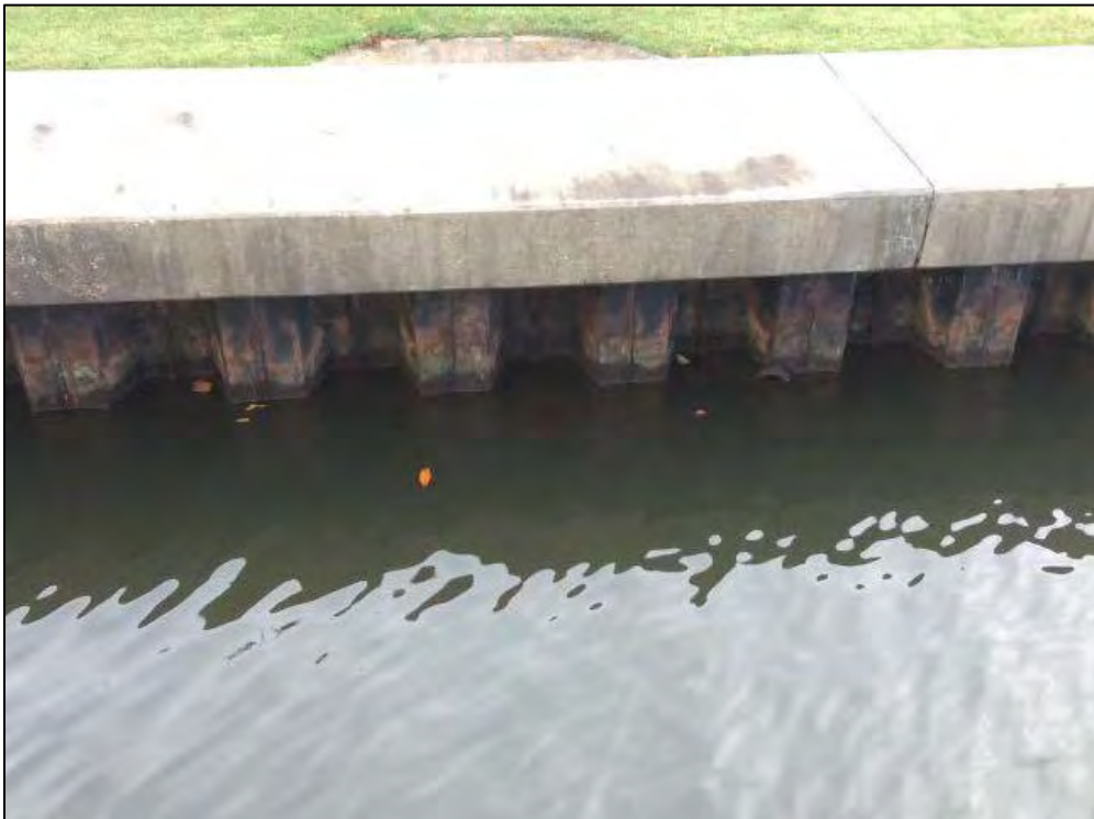
Figure 2-4 Example Sheet Pile Seawall Structure with Concrete Cap
