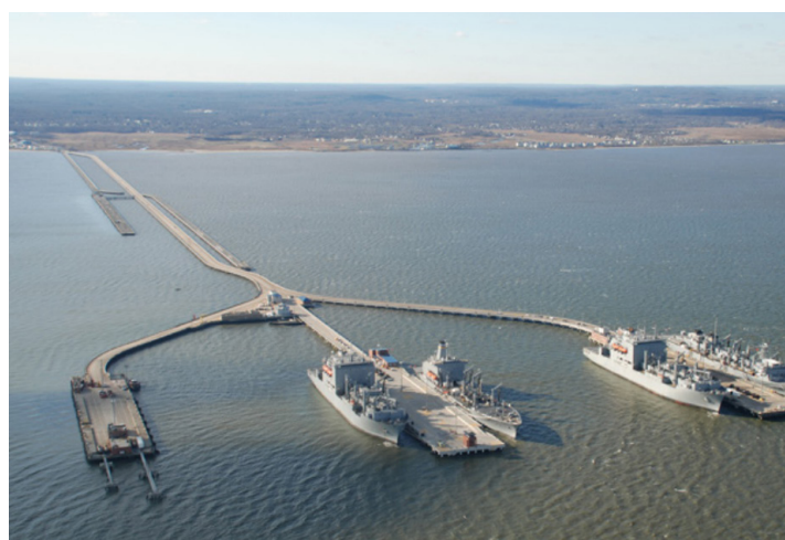
Ammunition Loading Pier Complex at NWS Earle.
