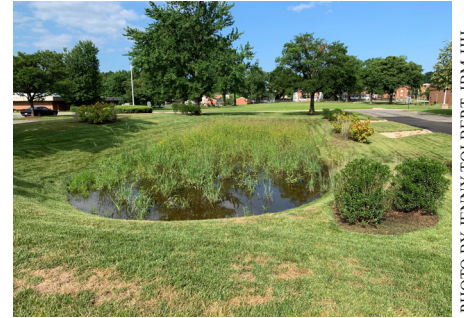
Figure 1. A bioretention area at Joint Base Myer-Henderson Hall (JBM-HH).
